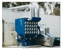
**DFO 4-48**Downflo® Oval cartridge collector on metal grinding.
