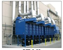
**DFT 4-48**Downflo® II cartridge collectors on metal spraying.
