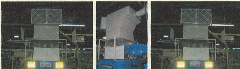
Three views of the Self-Contained Waste Removal System built by Industrial Metal Fabricators for the Winnipeg folding-carton plant.
